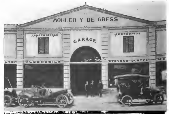
A Leading Garage in the City of Mexico.
